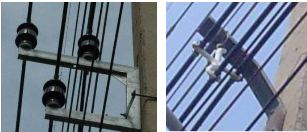
Figure 8: Installation of Pin & Post insulation (left) to replace a spacer (right).
